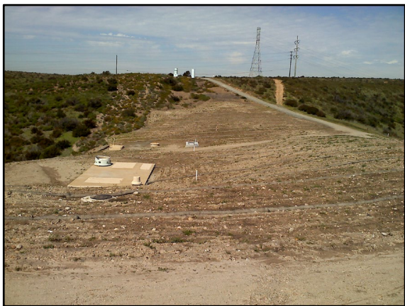
FRSII Site, After Construction
