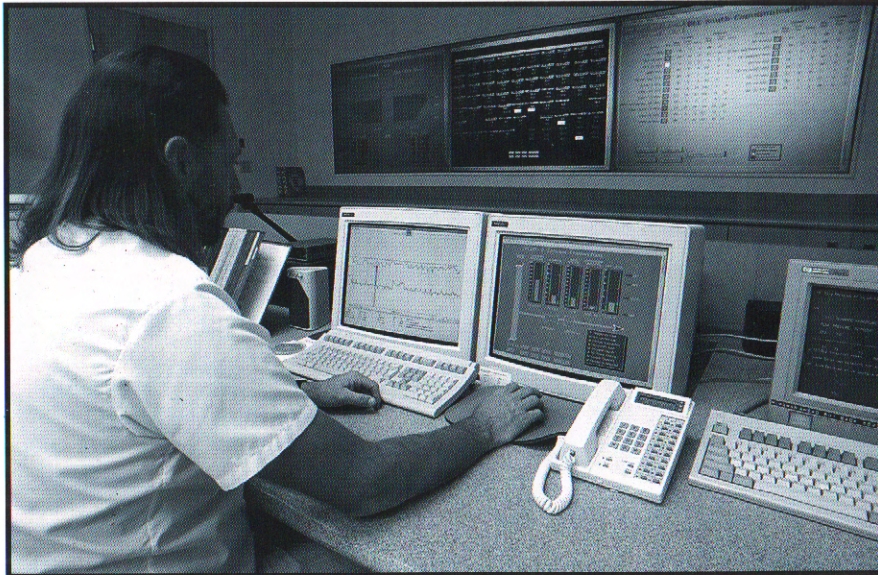
Operators regulate water deliveries to our member agencies from the control room in the Authority's Heilbron Operations Center in Escondido.
