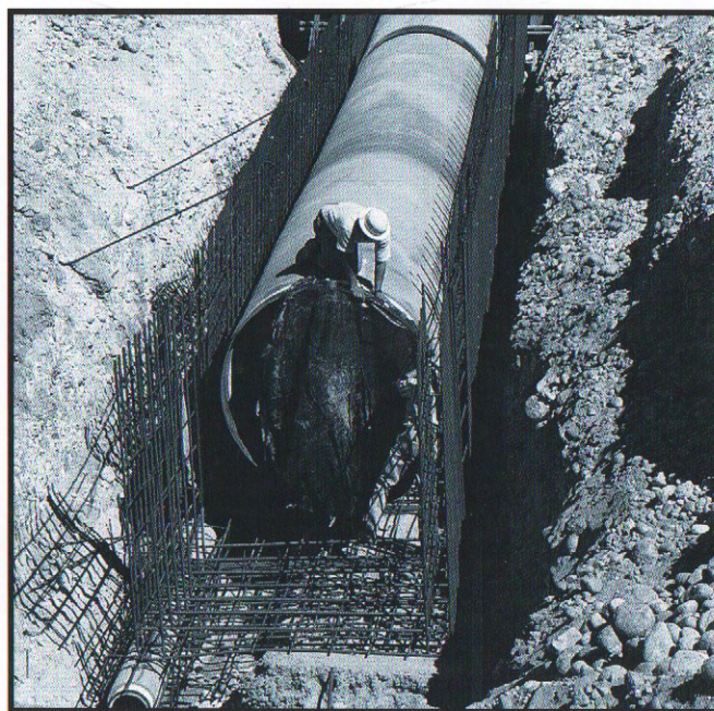
The Mission Trails Pipeline was completed and its Flow Regulatory neared completion. The pipeline will carry up to 240 million gallons of water a day, and the FRS—an underground reservoir—will help control water pressure.
