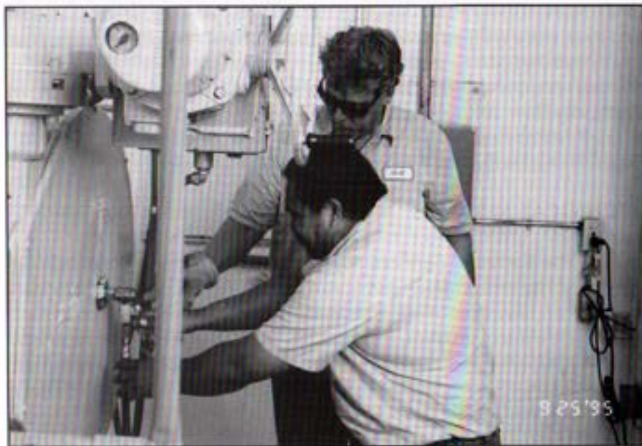
Senior Maintenance Specialist Mark Ancheta and Senior Maintenance Worker Scott Jensen servicing a flow control facility.
