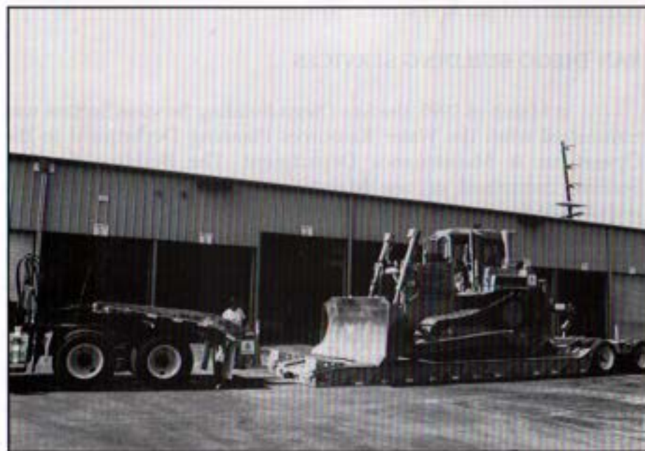
Maintenance Worker Ken Teter assists in loading a Caterpillar D6H dozer on to the new 40 ton low-bed equipment trailer.
