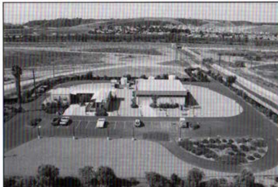
The City of Oceanside's 2-mgd Mission Desalter is the first brackish groundwater recovery project implemented by an Authority member agency.
