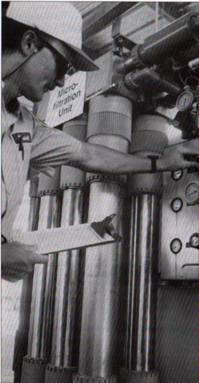
Microfiltration unit being tested at the City of San Diego's San Pasqual Advanced Water Treatment Facility. Union-Tribune/Tony Doubeck
