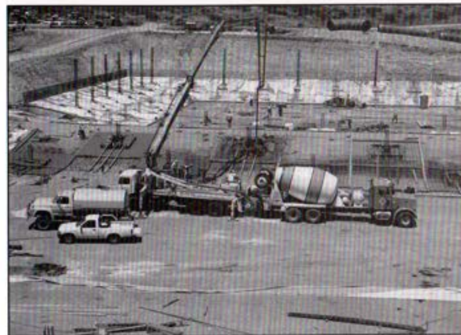
Placement of concrete floor slabs for flow regulatory structure.
