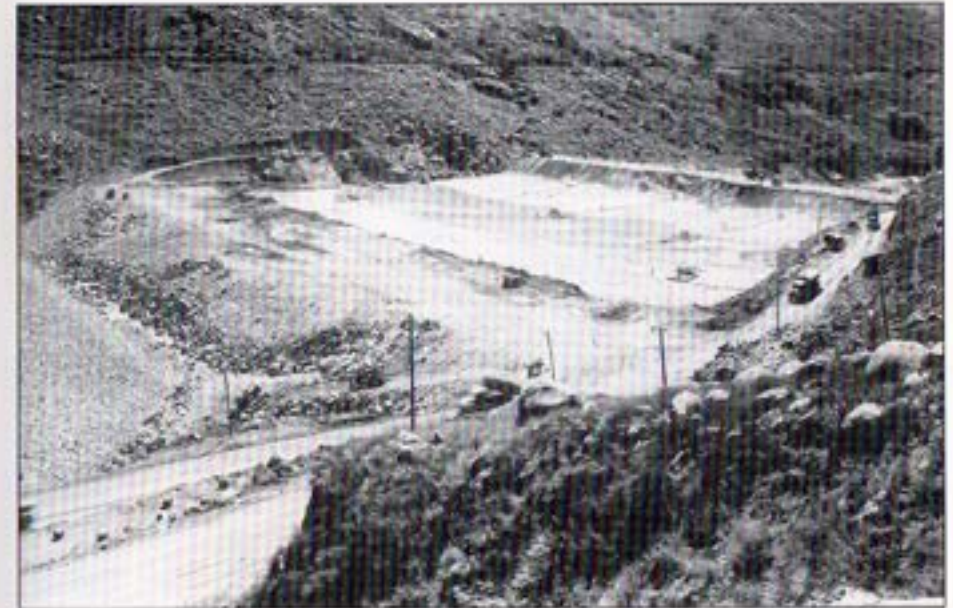
El Capitan Dam spillway under construction, circa 1933.
