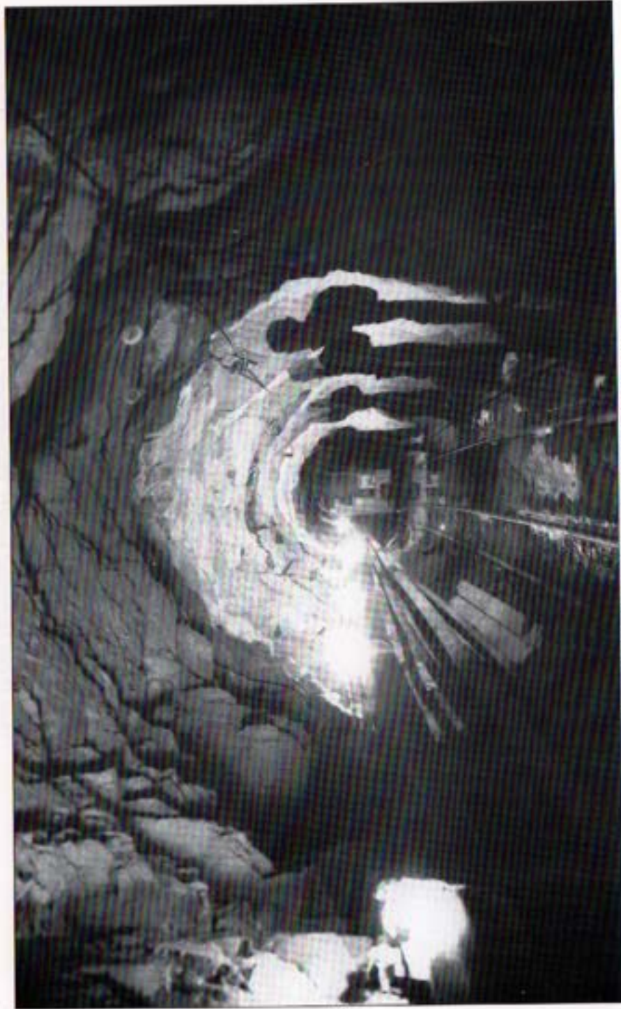
San Vicente Tunnel, San Diego Aqueduct, January 1946.
