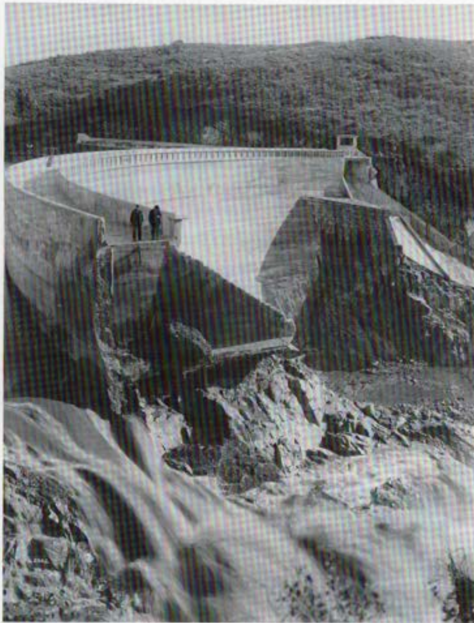
Sweetwater Dam break January 30, 1916. Reconstruction in 1917 included the addition of six siphon spillways on the north side to facilitate spilling. (San Diego Historical Society, Photograph Collection)
