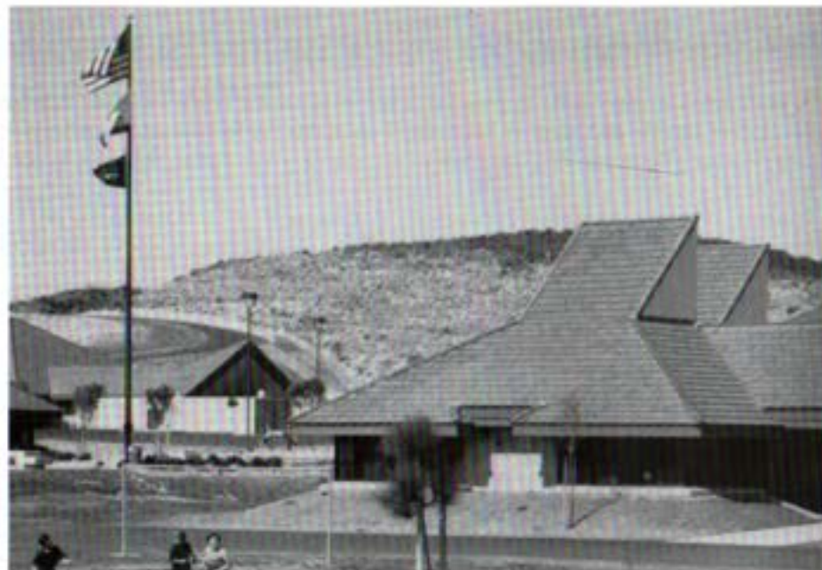
Aviara Oaks Elementary School is using reclaimed water provided by the Carlsbad Municipal Water District for landscape purposes.
