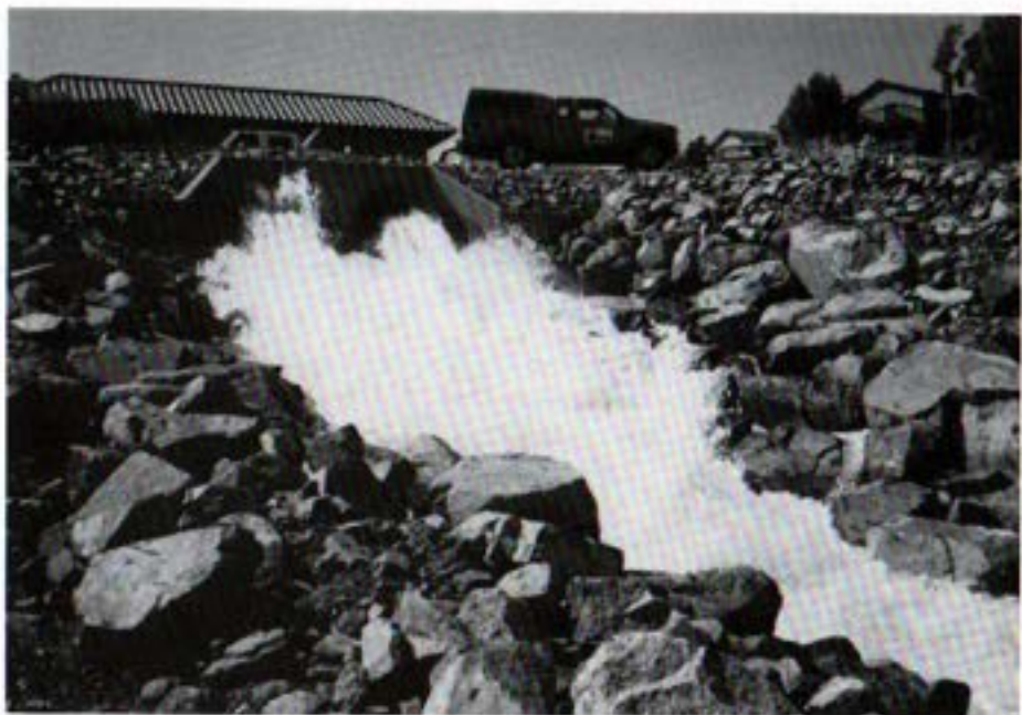
Water delivery from the flow control facility to the Sweetwater Reservoir
