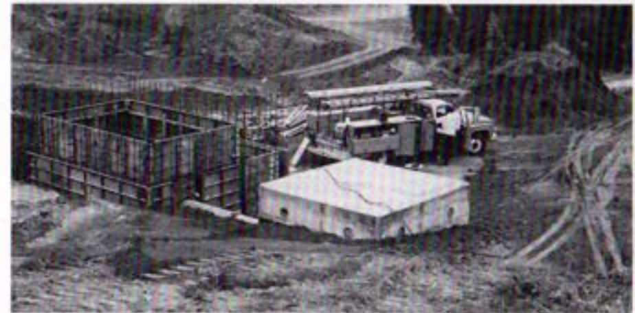
Bueno No. 10 service connection under construction by Water Authority forces.
