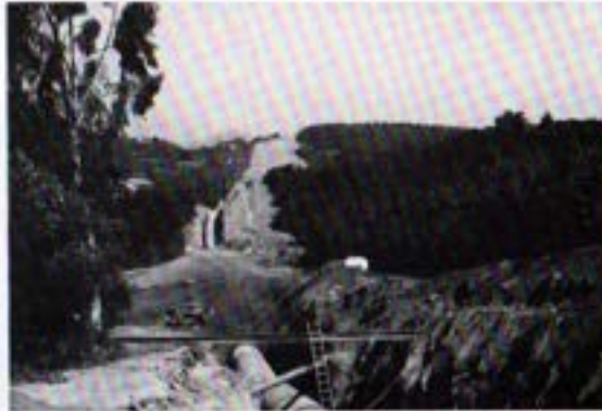
Backfill operation in Wilt Road, Pala Mesa area.
