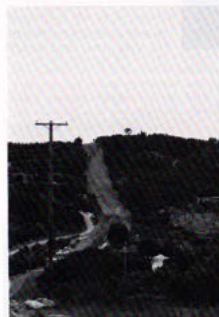
Pipe backfilled and finishing of the right-of-way in progress near Sumac Road.
