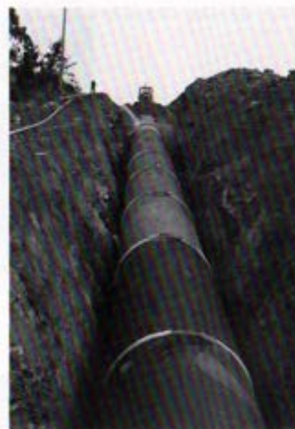
Backfilling 96-inch prestressed pipeline with sand in extremely rocky area.
