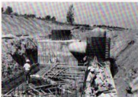
Pressure control structure and base of rejection tower under construction.
