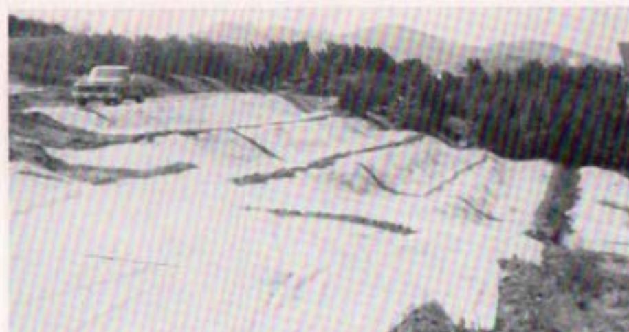
Avocado root-rot infestations on portions of the right of way require special treatment with gaseous methyl bromide applied to holes drilled to the infested depth and covered with plastic sheeting.
