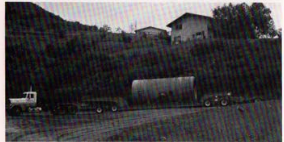
Prestressed concrete cylinder pipe sections 96-inch inside diameter by 22 feet long weigh 45 tons and require specially-built trailers to transport from pipe plant to the job site storage.
