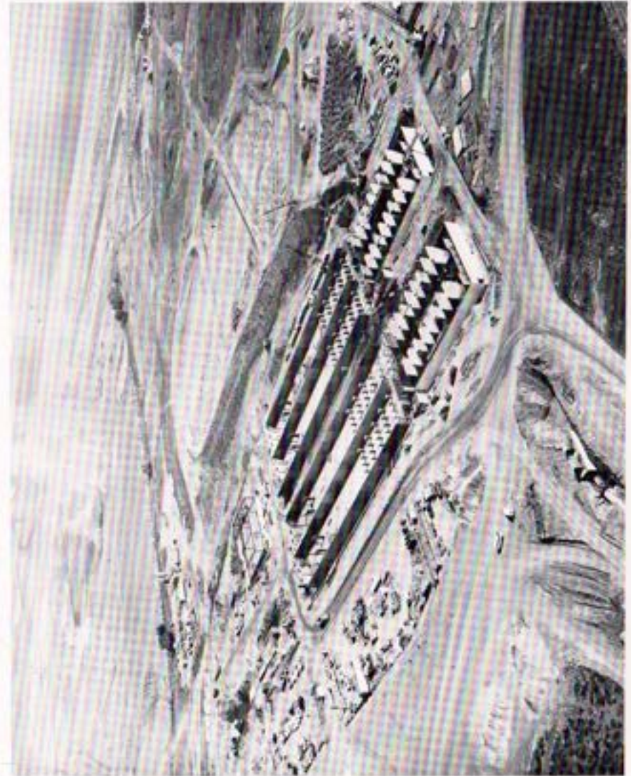
Robert A. Skinner Treatment Plant looking northeasterly towards Lake Skinner. Note dam in background. (Photo courtesy of Metropolitan Water District.)
