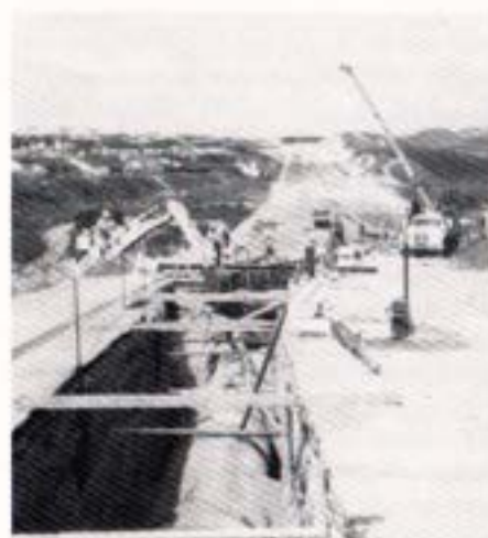
Pipe laying in Santo Road. Specification 224
