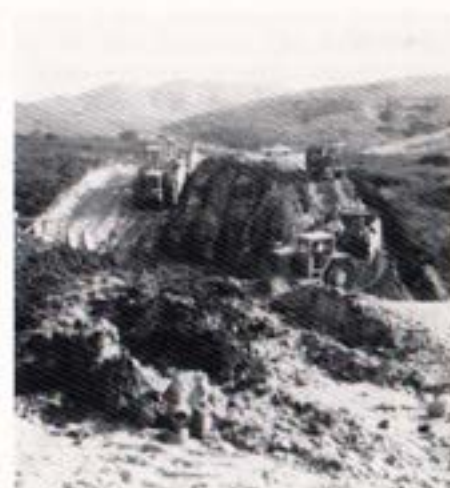
Trench excavation by motorized scrapers. Specification 224
