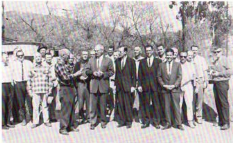
Member Agencies' Group Inspecting Cross-Connection
