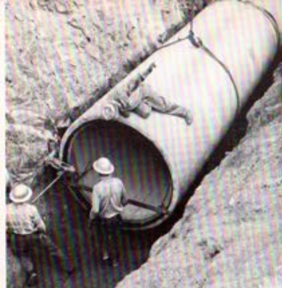
Laying 60 inch Prestressed Concrete Pipe
