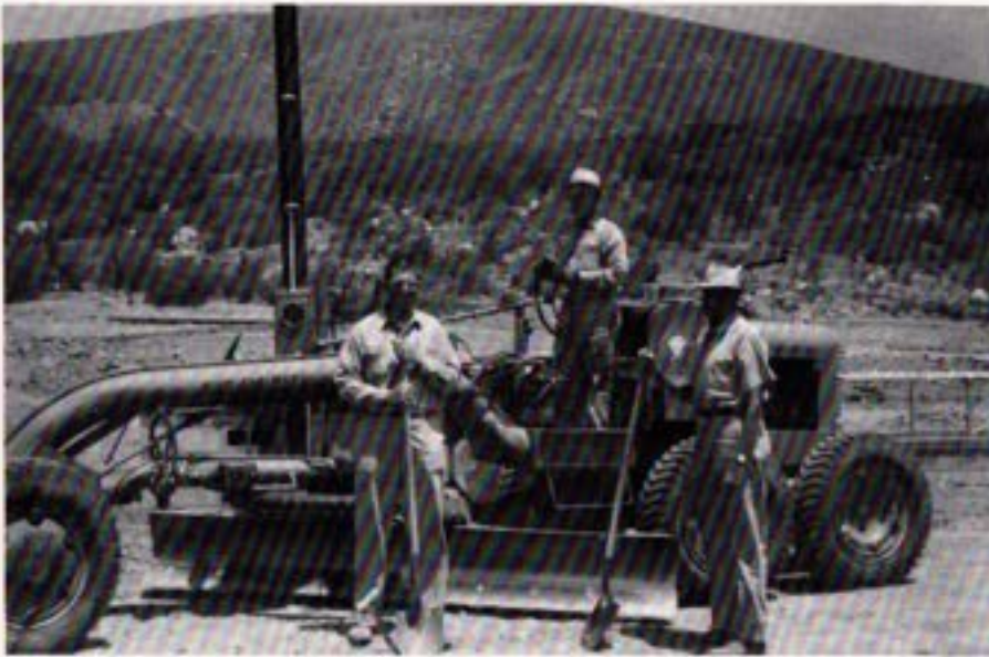
Road Grader Crew
