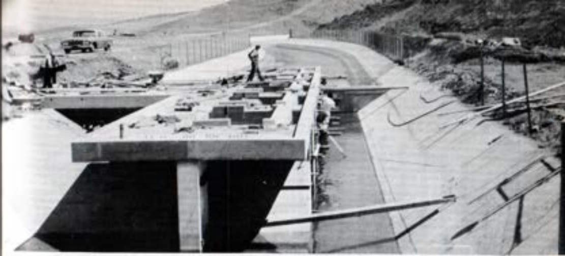
Platform for Screens at End of Second Aqueduct Canal
