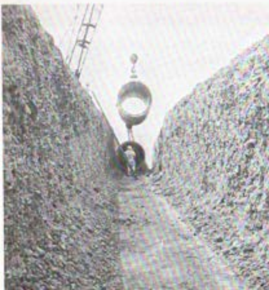
Pipe Laying on Second Aqueduct
