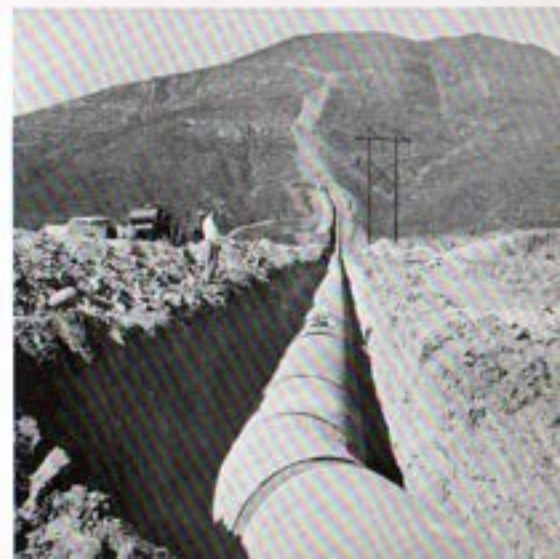
Second Aqueduct Activities
