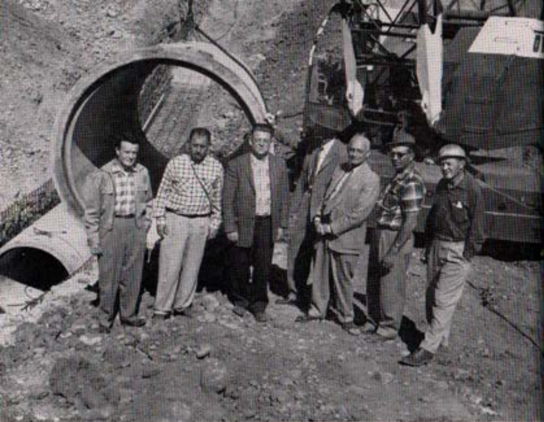
Laying First Pipe in Lake Murray Crossing
