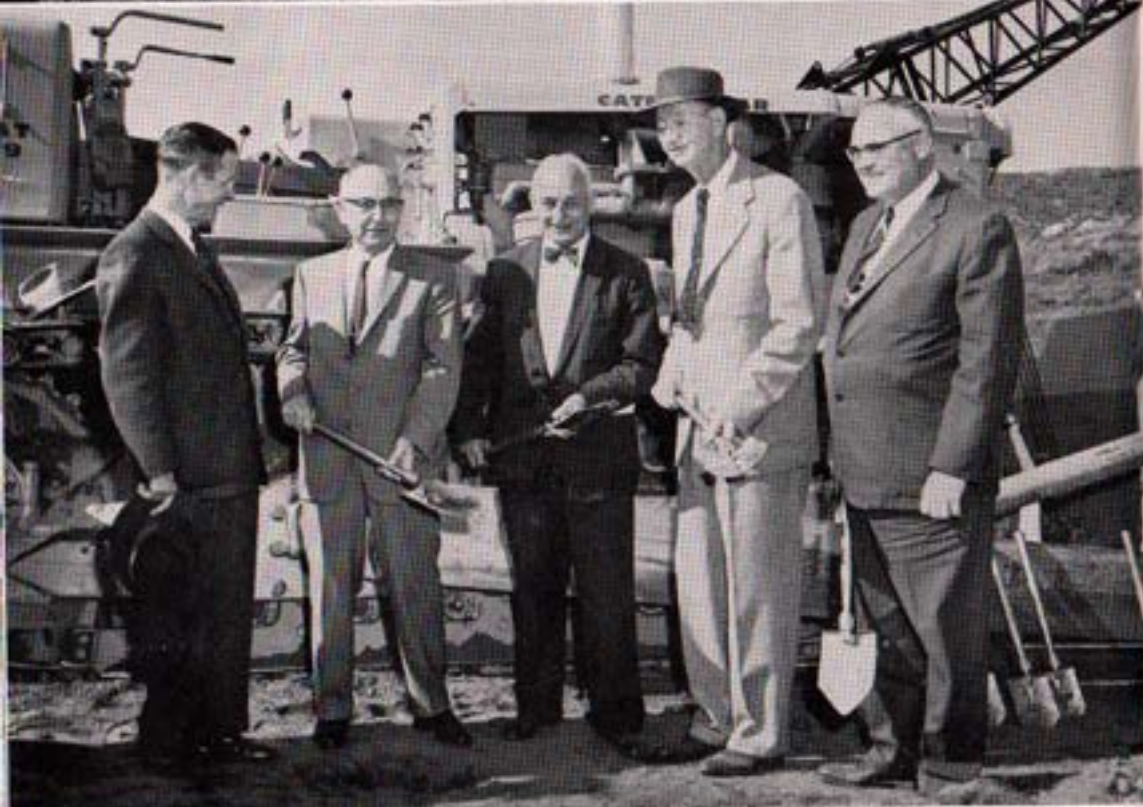
Metropolitan Water District Section of Second Aqueduct
