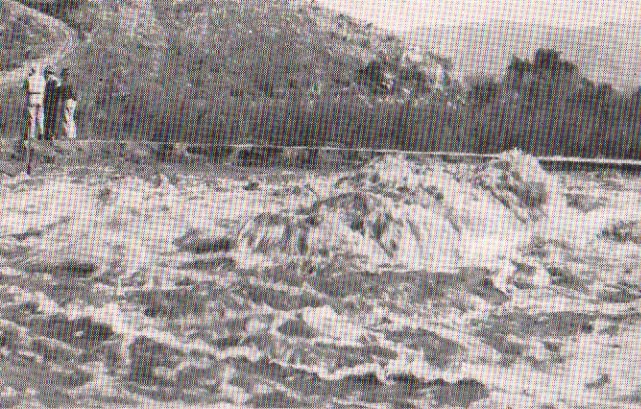
Colorado River water gushing from break in Second Barrel on San Luis Rey River crossing.
