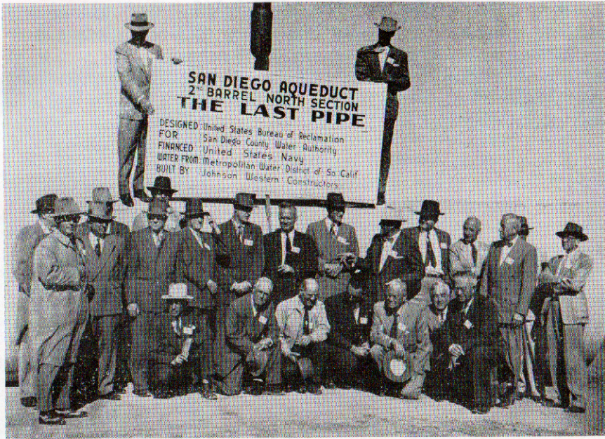
Gathering at placing of last pipe.
