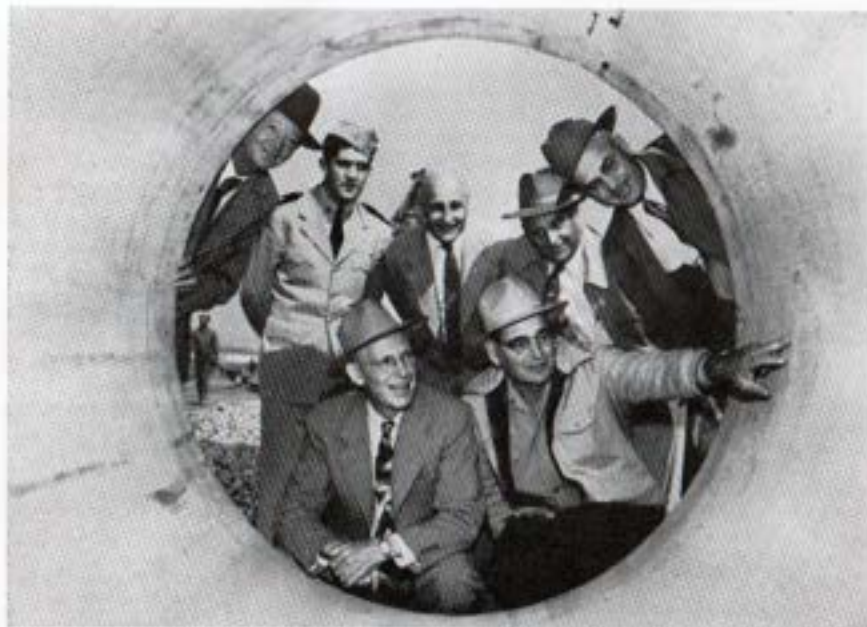
Inspection of First Pipe of Second Barrel of San Diego Aqueduct by Representatives of U. S. Bureau of Reclamation, Contractors, and the Authority
