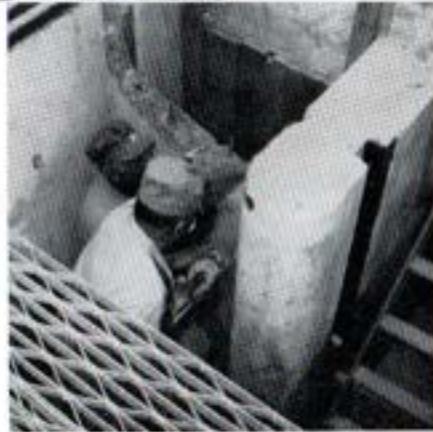
Miscellaneous Maintenance Activities of Authority Personnel
