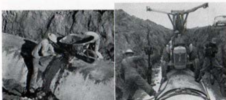
Filling Pipe Joints with Cement Mortar.
