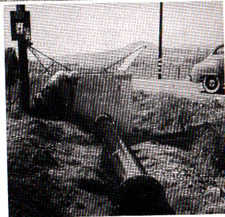
Installation of Orifice Pipe at Sta 1121+70 for metering of temporary supply to Vista Irrigation District.
