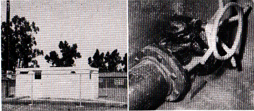
View of Plug Valve in sub-structure
