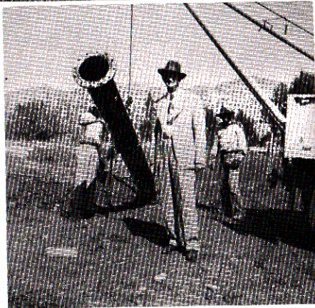
Chairman Heilbron inspecting Orifice pipe.
