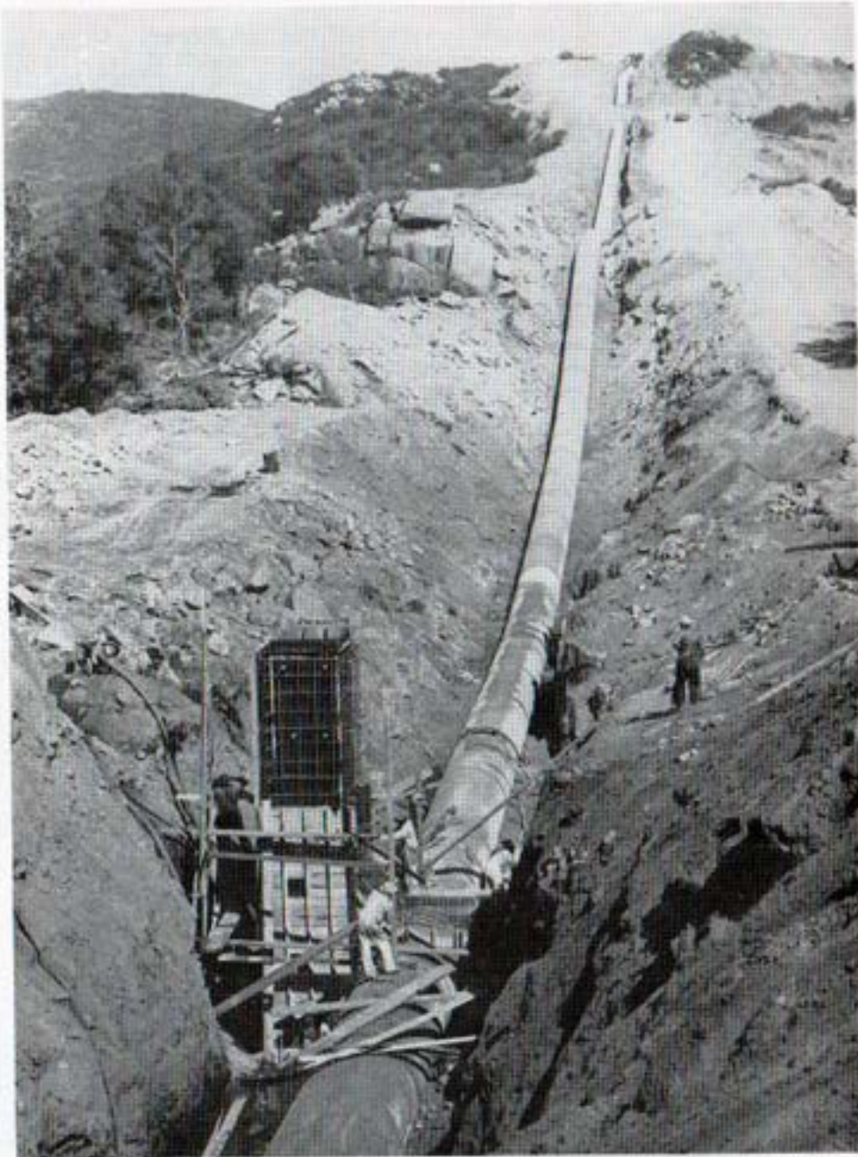
Construction of First Barrel North of Oat Hill Tunnel
