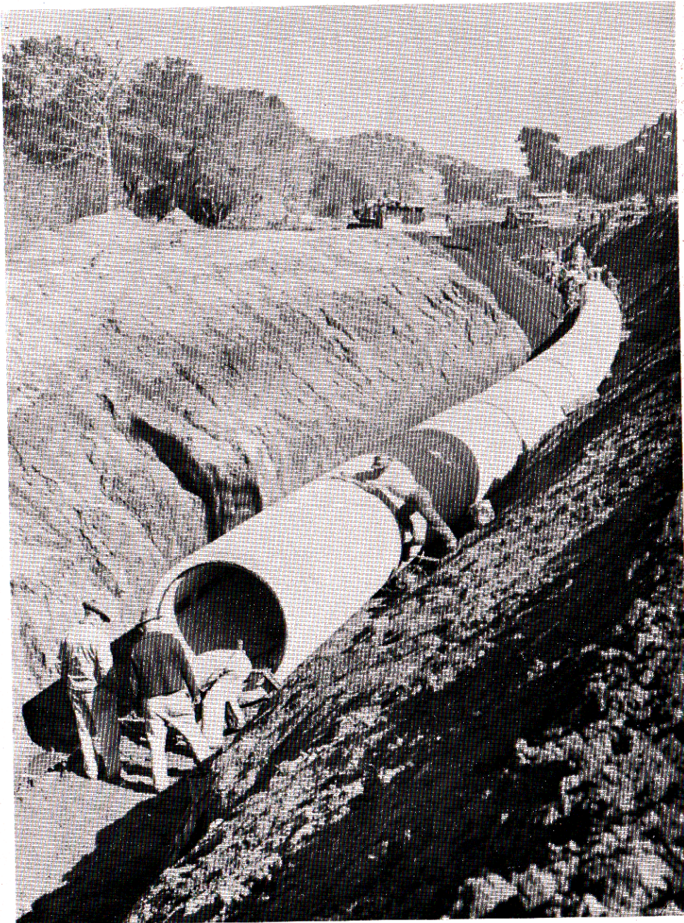
Constructing first barrel of Aqueduct near Temecula
