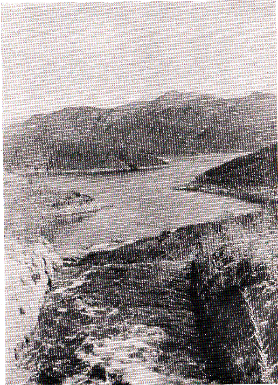
End of San Diego Aqueduct, showing water discharging into San Vicente Reservoir
