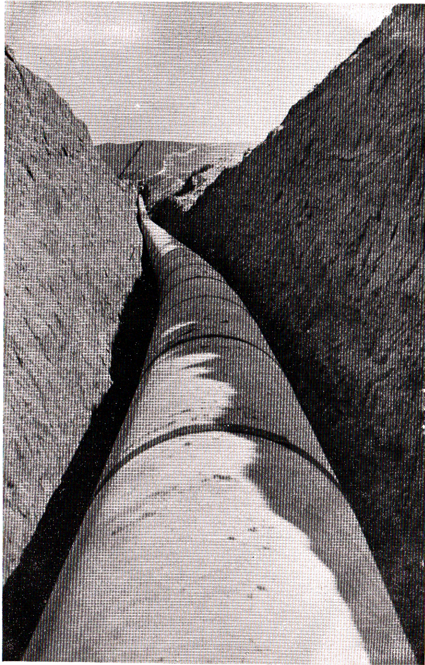
Aqueduct pipe in place.
