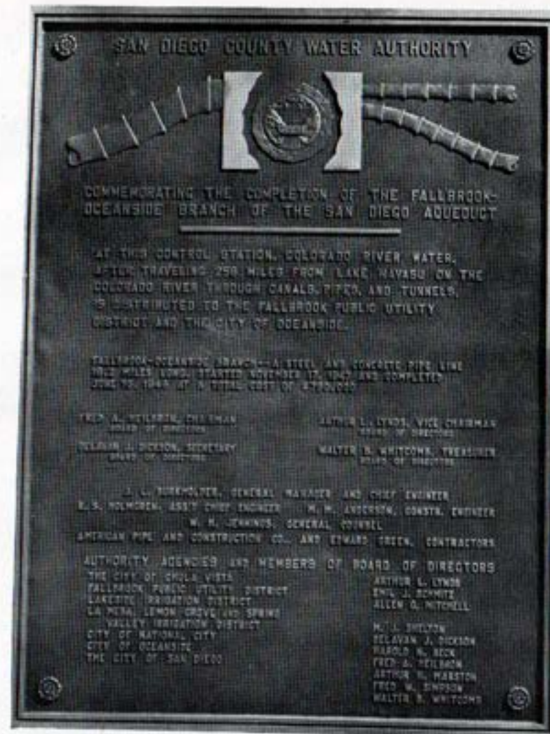
Bronze tablet at Fallbrook Control Station.
