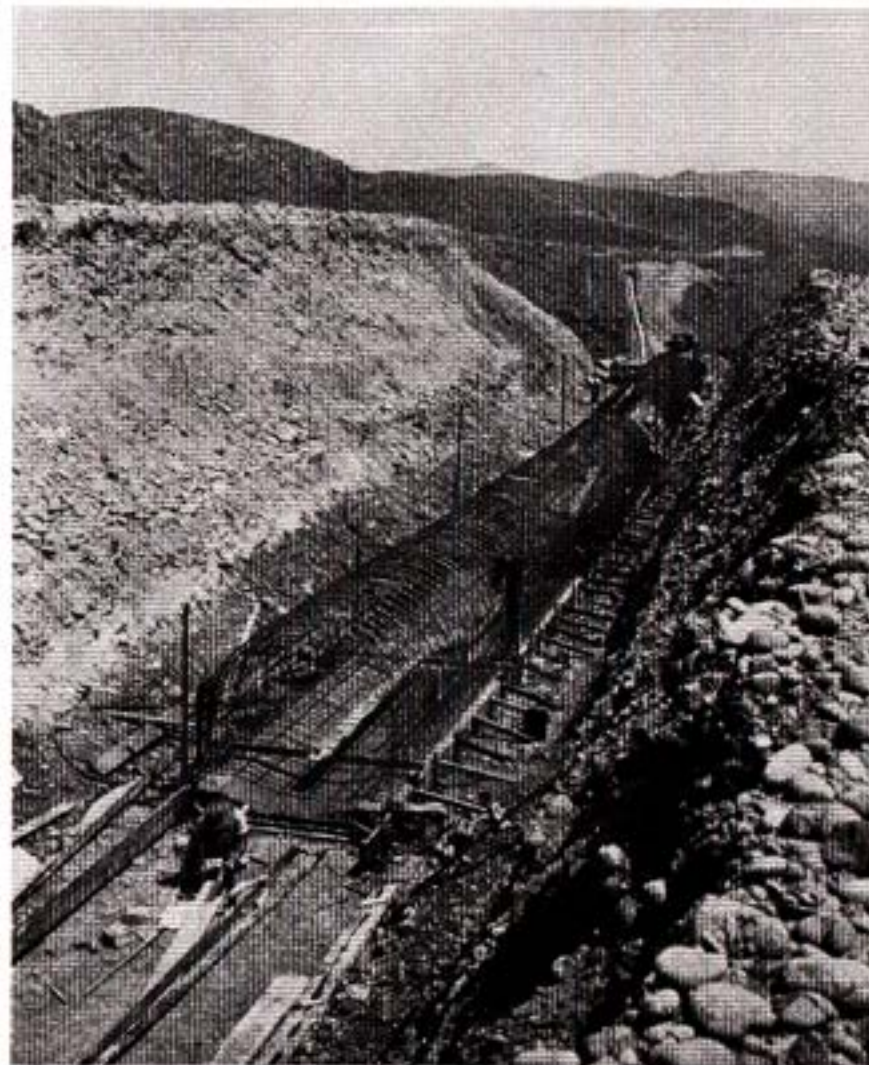
Cut-and-cover section, Southerly end of Fire Hill Tunnel, San Diego Aqueduct.
