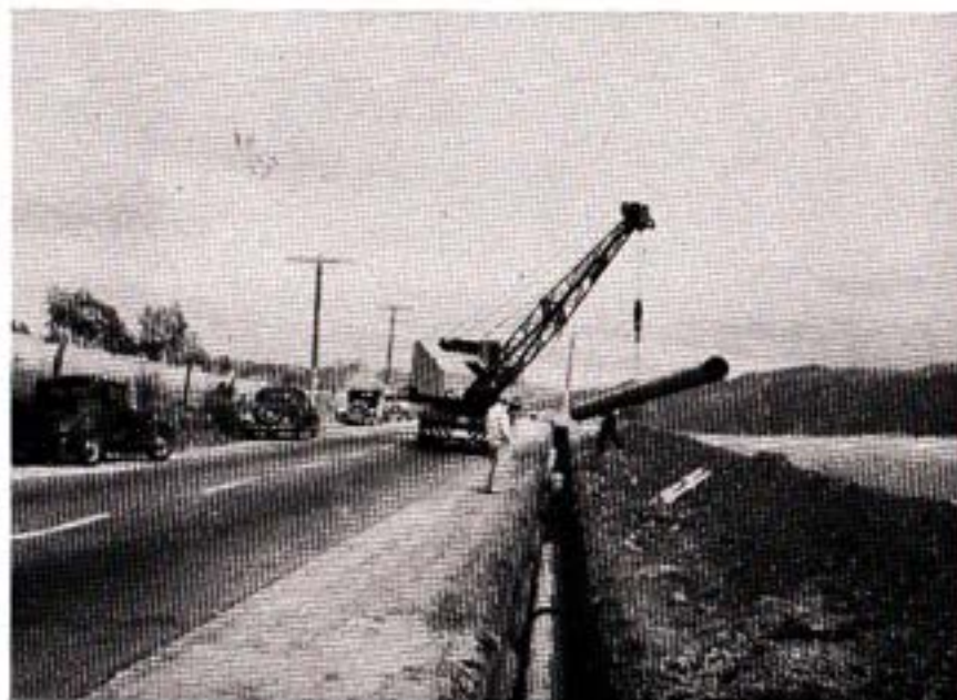
Fallbrook-Oceanside Branch—Laying Pipe along U.S. Highway No. 395.
