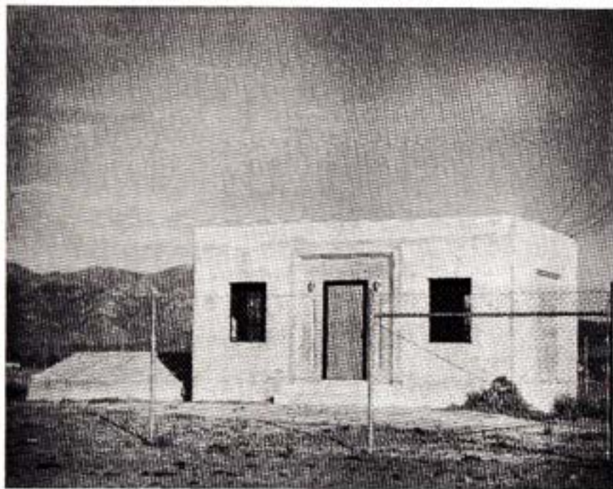
Lakeside control station.
