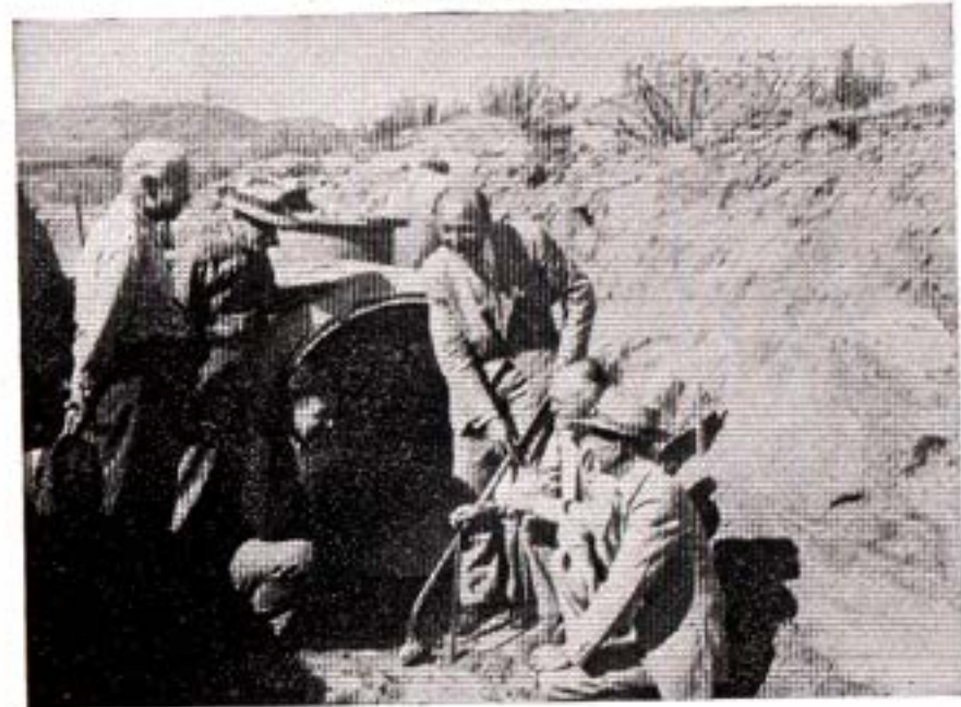
La Mesa-Sweetwater Extension—Laying first pipe on Sept. 18, 1947
