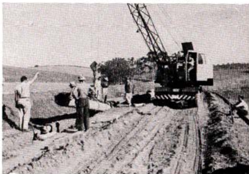
Fallbrook-Oceanside Branch—Laying first pipe Jan. 9, 1948.
