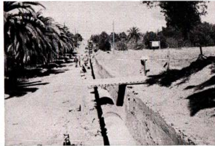
La Mesa-Sweetwater Extension—Laying pipe along Hillside Drive—Station 200.
