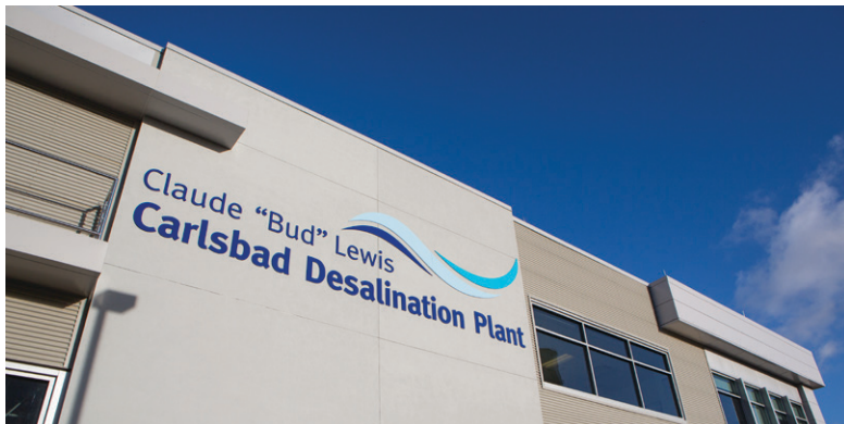
The Carlsbad Desalination Plant began operations in 2015.
