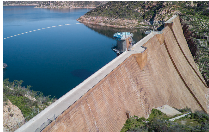
Today , San Vicente holds more than double of the reservoir's original capacity.
