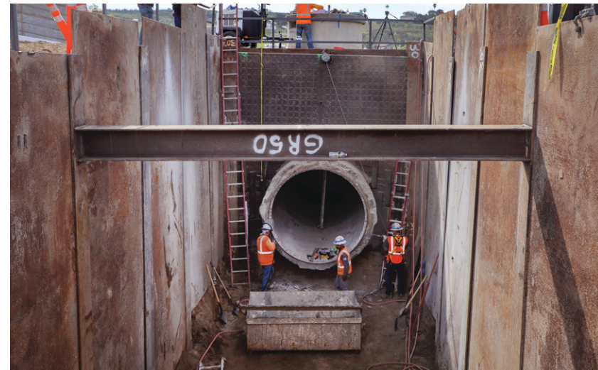
An urgent repair on Pipeline 4 (2022)
