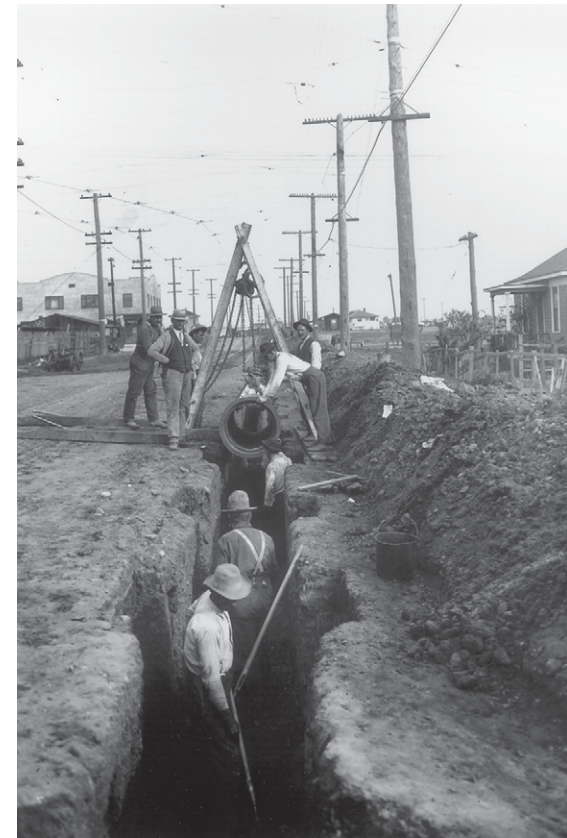
Laying water pipe (1911)
