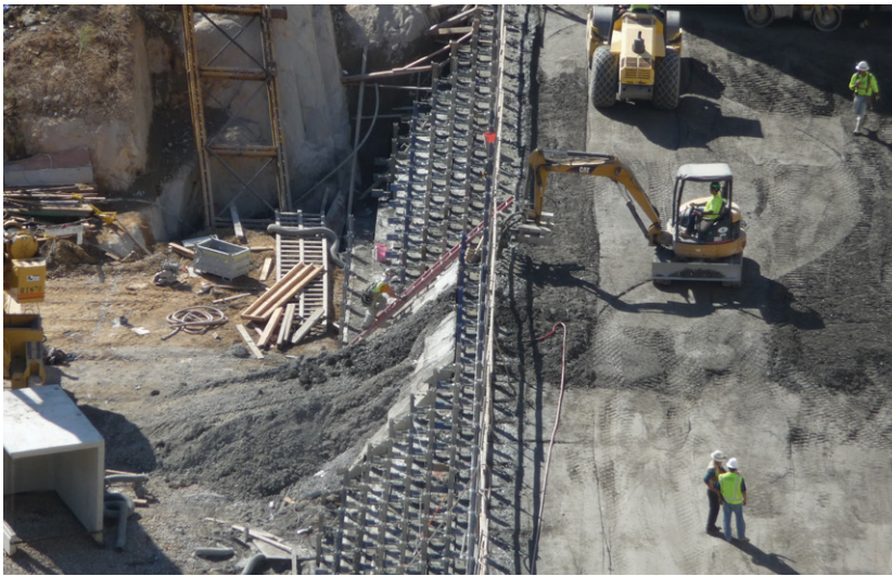
Construction of the San Vicente Dam Raise began in 2009.
