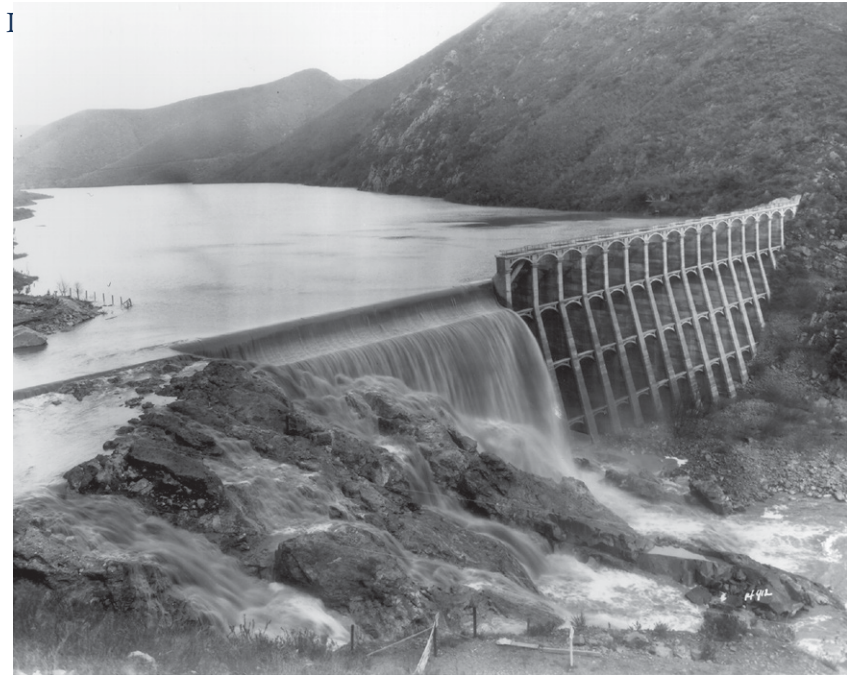
Lake Hodges Dam with spillway (c. 1920)
