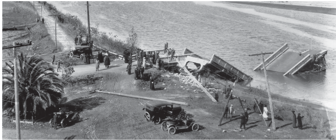
Damaged bridge at Old Town after the 1916 flood
