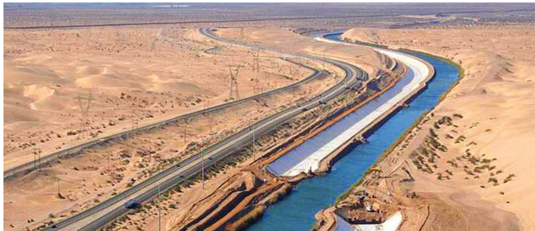
Concrete lining the All-American Canal prevented huge amounts of water from disappearing in to the desert sand.
