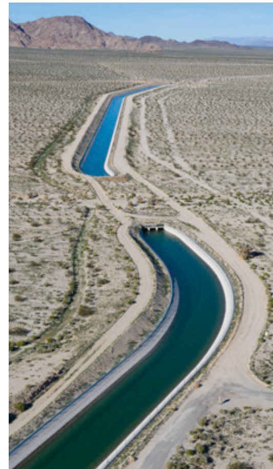
Colorado River Aqueduct
