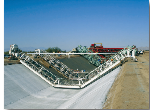
The Water Authority has secured additional Colorado River supplies through canal-lining projects.
