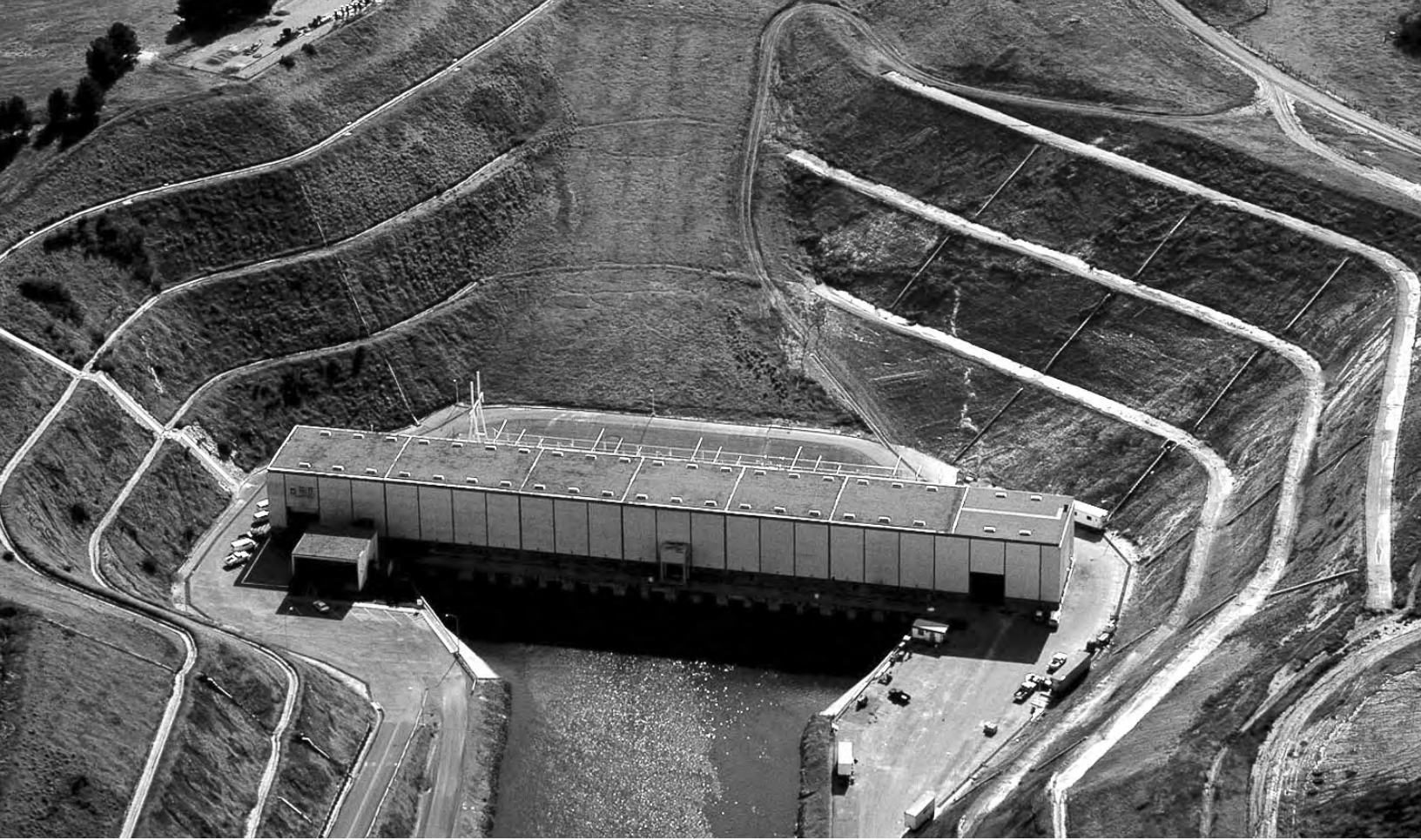
The State Water Project's Harvey O. Banks pumping plant pushes water into the 444-mile California Aqueduct for delivery to Southern California
