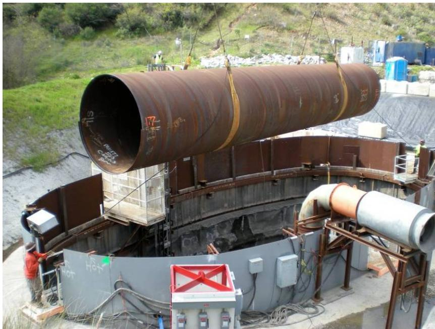
50-foot-long pipe segments being lowered into the tunnel.
