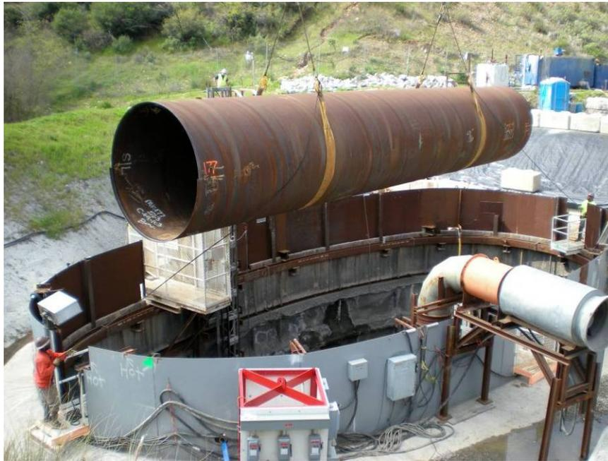
*50-foot-long pipe segments being lowered into the tunnel for the San Vicente Pipeline.*
