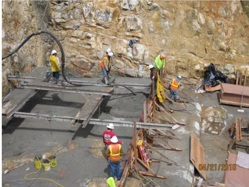
*The first phase of the construction included excavating the foundation of the dam and then placing concrete to shape and prepare the foundation for the new concrete that will raise the height of the dam.*
