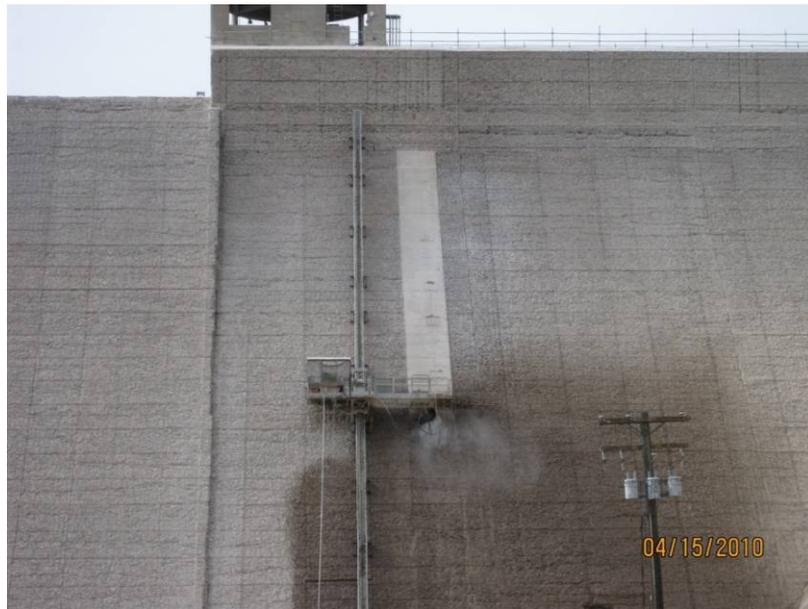
*The contractor has completed hydrodemolition, which removed about two inches from the surface of the dam to prepare it for the new concrete.*
