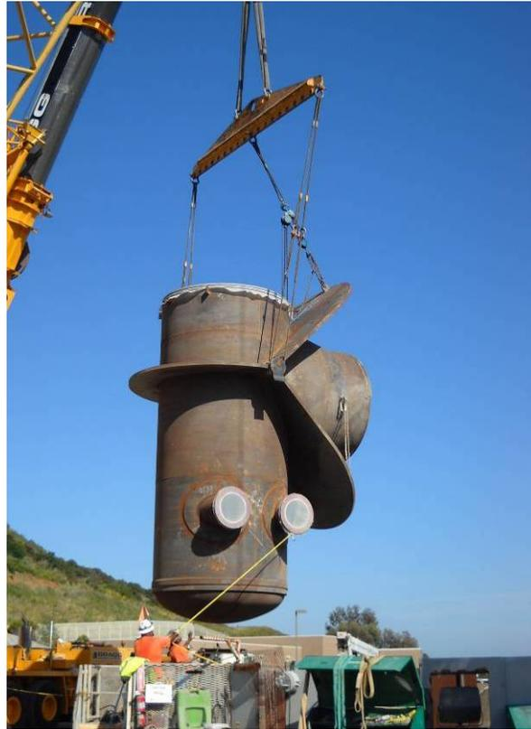
*In May, crews lowered this riser pipe down into the tunnel at the West Shaft. The two smaller openings on the side of the riser pipe will turn up and extend to the surface serving as drain lines.*
