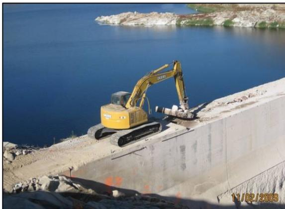
*The contractor removed the top one foot of concrete from the dam to help the new concrete bond to the existing dam.*
