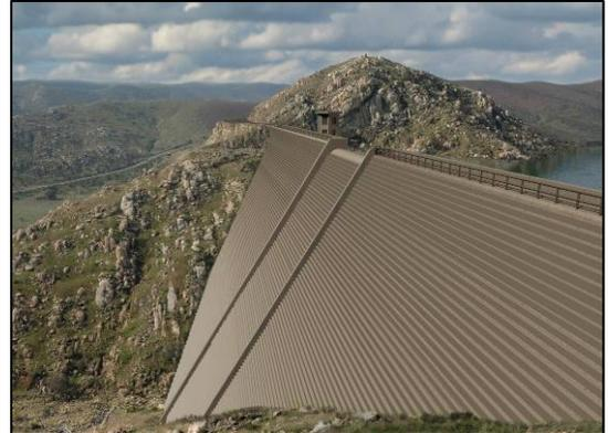
*A rendering of the future dam shows the stair-stepped appearance of the roller-compacted concrete.*
