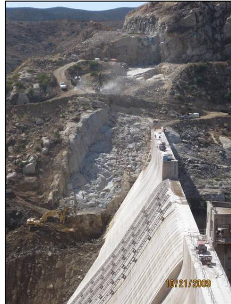
*The excavation on the hill shows how tall the raised dam will be – the tallest dam raise in the country.*
