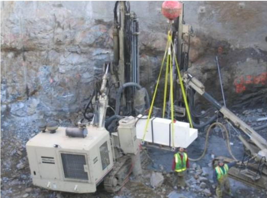
Drilling equipment inside the pump station pit is used to drill holes in the rock.
