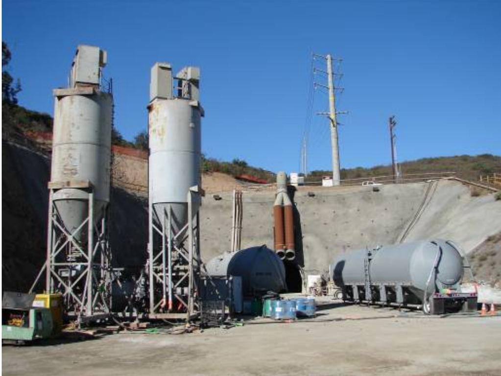
Cellular grout mix batch plant equipment (used to make the grout, which is then pumped into the tunnel to seal the area between the tunnel and the pipe).
