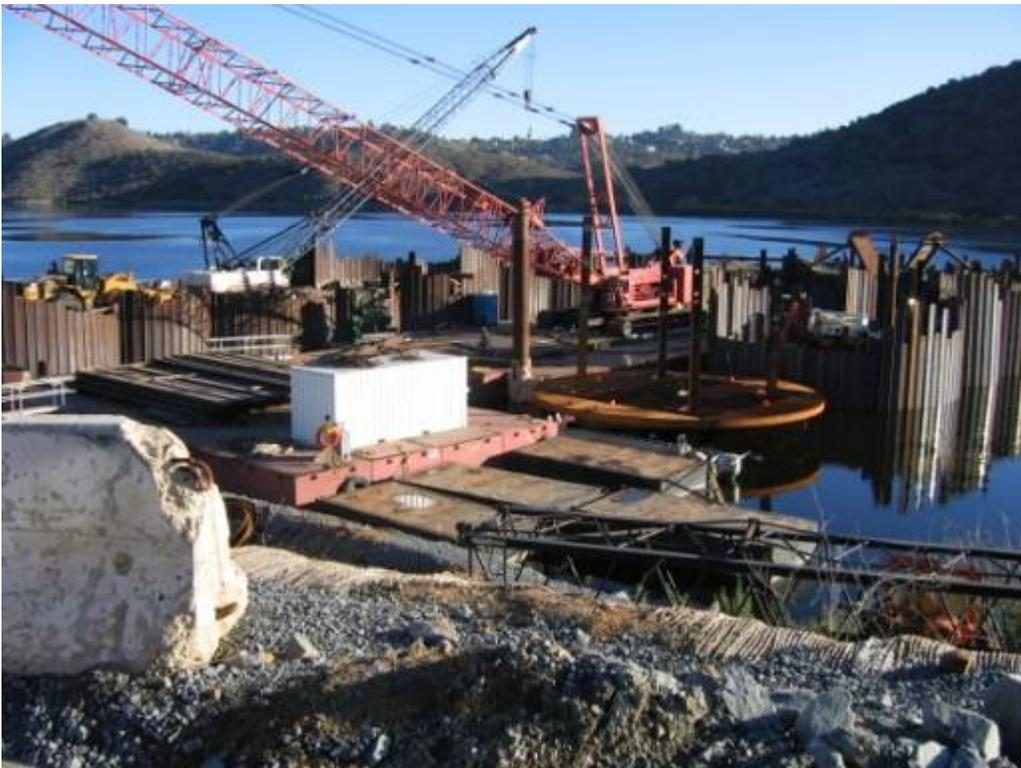
Cofferdam construction is nearly complete. Once it is done, the water will be pumped out, and then construction will begin on the inlet-outlet structure.
