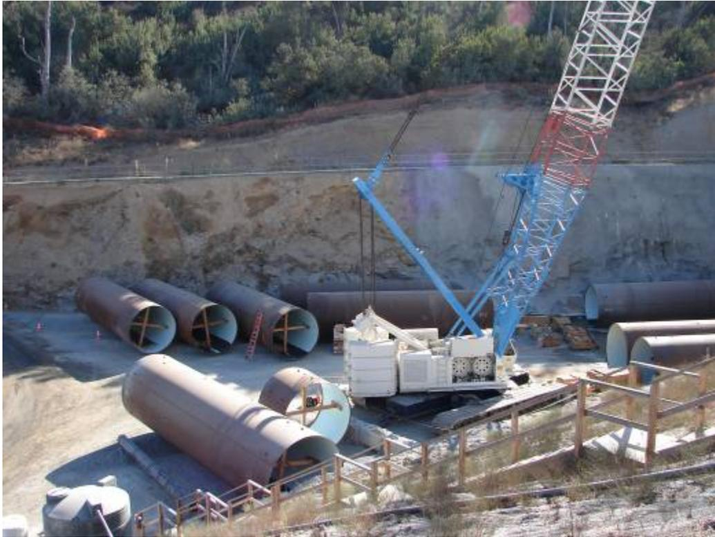
Steel pipe segments to be installed in the tunnel (each one is 40 feet long).
