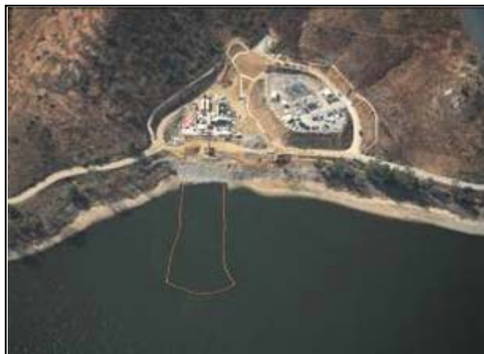
The cofferdam has been removed and orange buoys mark the area above the inlet-outlet structure.
