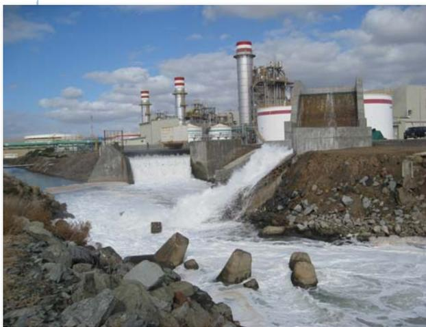
*A binational seawater desalination project in Rosarito Beach might use this existing water intake facility for a local electric power plant as a source of ocean water for treatment.*
