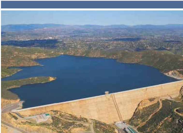
The regional surface water yield is supported by 24 surface reservoirs. The Olivenhain Reservoir, completed in 2003, is the region's newest reservoir.
