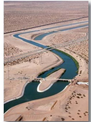
Water conserved by the All-American Canal Lining Project is an important part of the Water Authority's Colorado River water transfer supplies.
