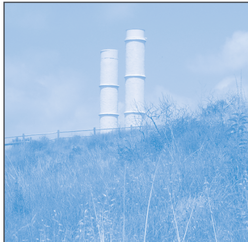
New facilities will eliminate the need for most of the blue vent stacks on hilltops in Mission Trails Regional Park.
