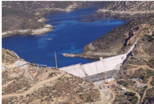
San Vicente Dam Raise
