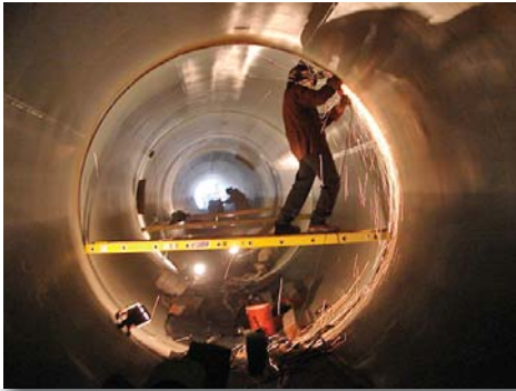
Welding the Lake Hodges Pipeline
