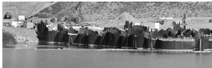
The temporary cofferdam holds back water while the inlet-outlet structure is built.
