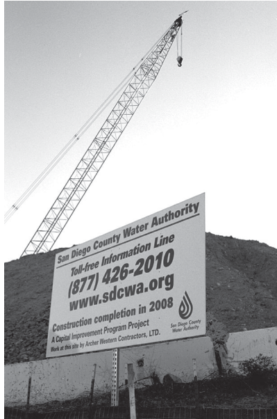
Construction activity can be seen from Interstate 15.
