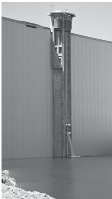
Imported water cascades into the Olivenhain Reservoir.
