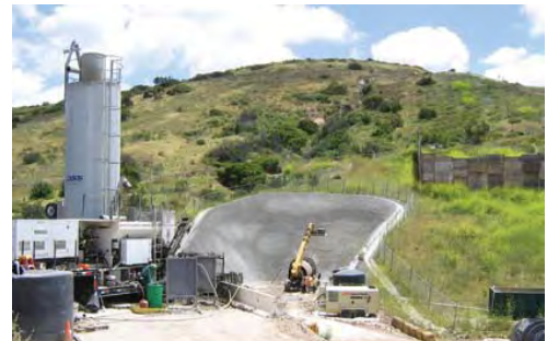
Inlet Tunnel Portal, Mission Trails Pipeline, 2010
