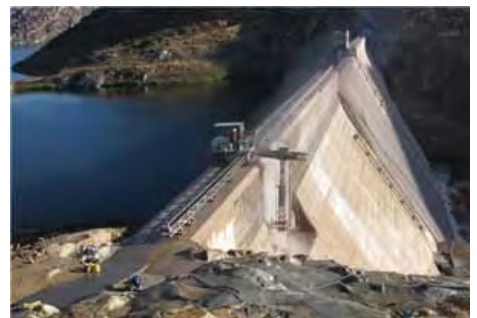
Construction on the San Vicente Dam Raise, 2010
