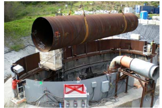
Large 50-foot-long pipe sections will create the San Vicente Pipeline.
